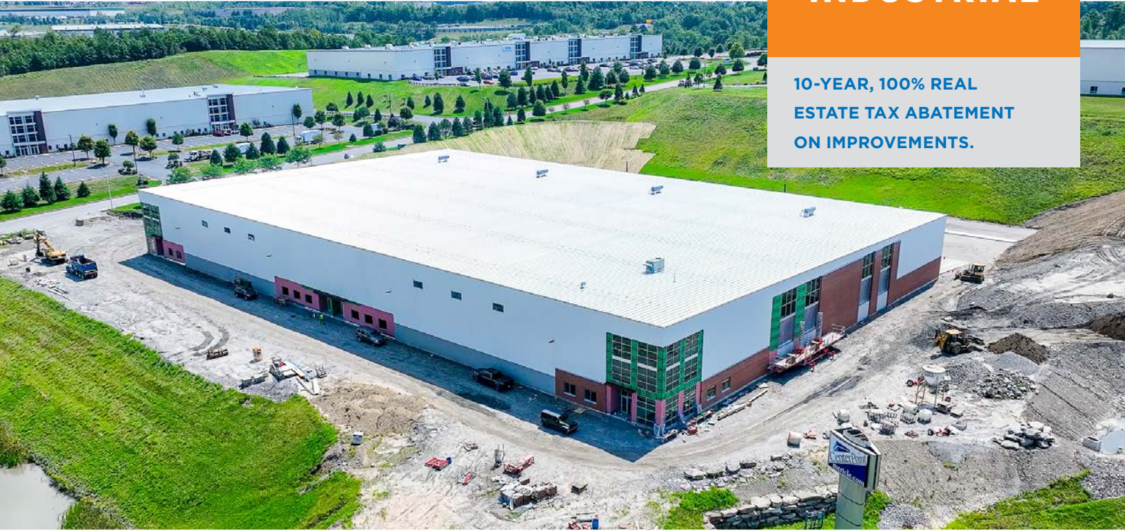
AUGUST CONSTRUCTION PROGRESS PHOTOS
