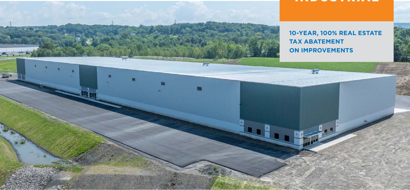
AUGUST 2024 CONSTRUCTION PROGRESS PHOTOS
